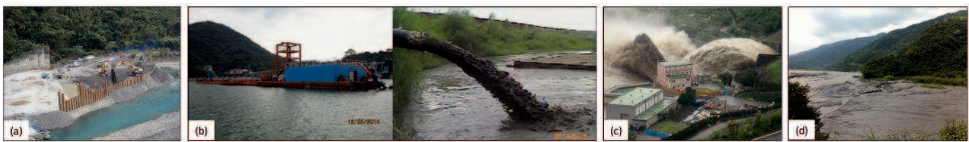
Figure 4. Sediment management strategies in Taiwan [5] : (a) mechanical dredging from a sabo dam in Yixing, Shihmen basin, (b) hydraulic dredging at Shihmen reservoir (photo courtesy of WRA), (c) Sluicing at Shihmen Reservoir during Typhoon Soulik in 2013 (WRA), (d) Drawdown flushing at Wujie Reservoir
