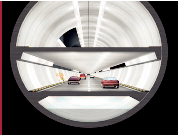
Dual deck motorway tunnel concept
