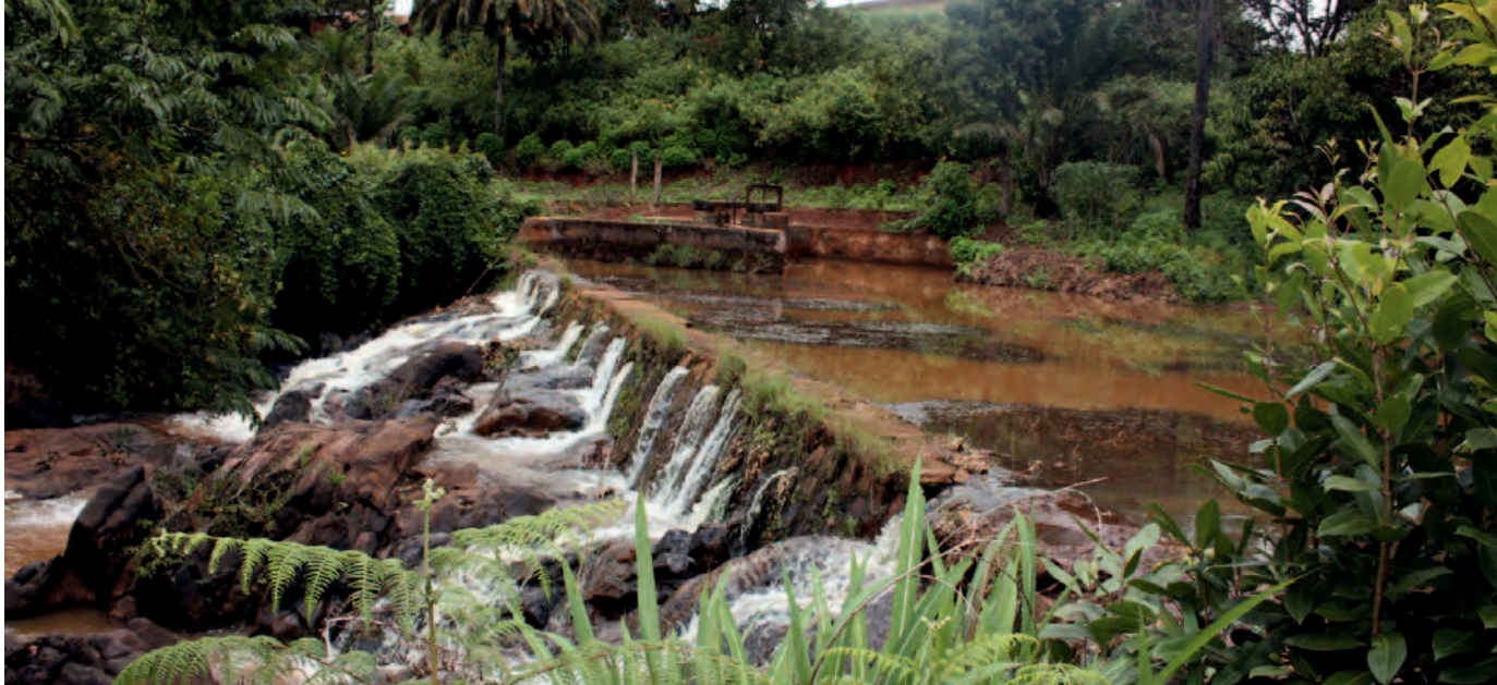
Figure 2 - View onto the existing weir from downstream and overhaul measures
