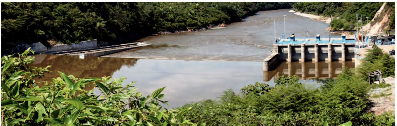
Figure 1. Intake of the Saldaña River; Tolima Triangle irrigation project, Colombia
