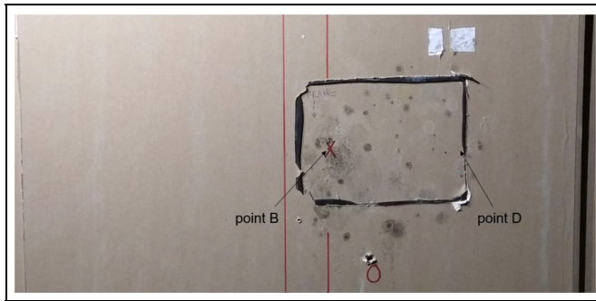
Figure 8. Mold growth was observed on the interior face of the EGS after the MCONI test. The wood frame was located between the vertical lines, the inlet pipe was located opposite the spot marked with the letter “X,” and the outlet hole was located next to the letter “O.” The black ethylene propylene diene monomer (EPDM) sealant is visible at the edges of the EGS piece, whose outer surface was additionally taped. The EGS piece was removed at the end of Phase 3 for probe installations. The board was kept intact before that point.
