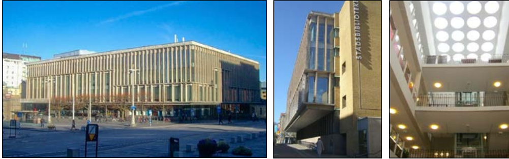
Figure 9, 10 and 11. The original facade seen from inside. To the left, the brick façade seen in the corridor at the ground floor. In the middle the café in the extension at the second floor seen from the third floor. To the right, stairs to the third floor. Photography: Magnus Rönn, 2020.
