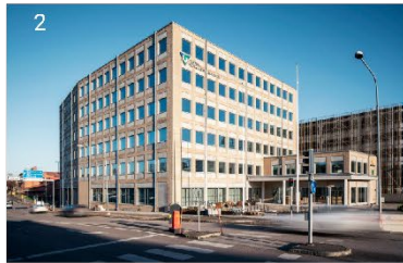
2 Facade of Case S.
