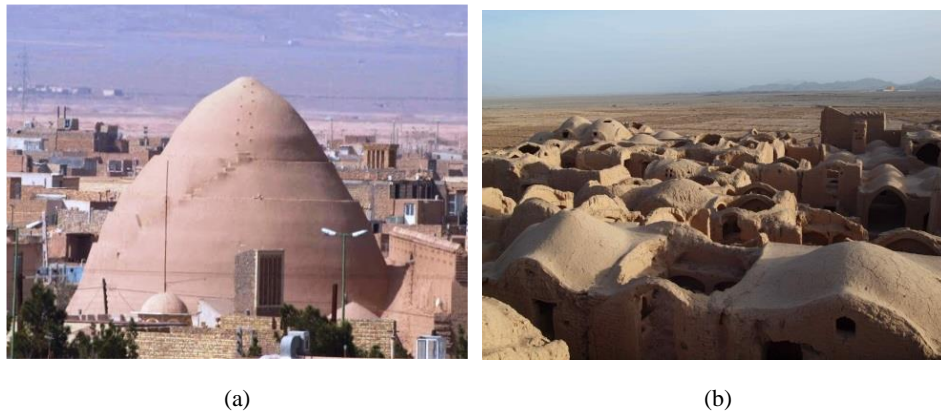
Figure 1 Examples of domes in the Iranian architecture, (a) typical Central-Asia icehouse (b) traditional house made of adobe bricks in Yazd, Iran (see online version for colours)
