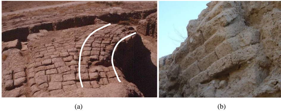
Figure 6 (a) Brick layout at the base of the Round Hall (the white lines indicate the expected base of the dome) (b) Brickworks at the impost of the vaulted covering placed over the north-west access of the Round Hall, with bricks arranged along inclined courses (see online version for colours)
