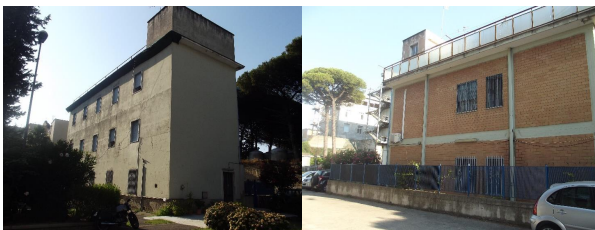
Fig. (5). Photos of the [NB] building.
