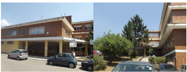
Fig. (4). Photos of the [AB] building.
