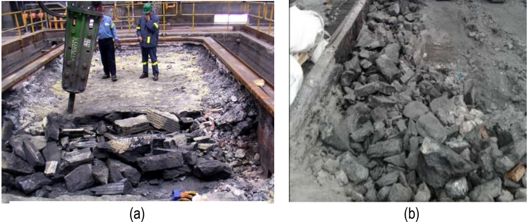
Figure 1-10. (a) Demolition of SPL [92], (b) SPL after breaking up [94].
