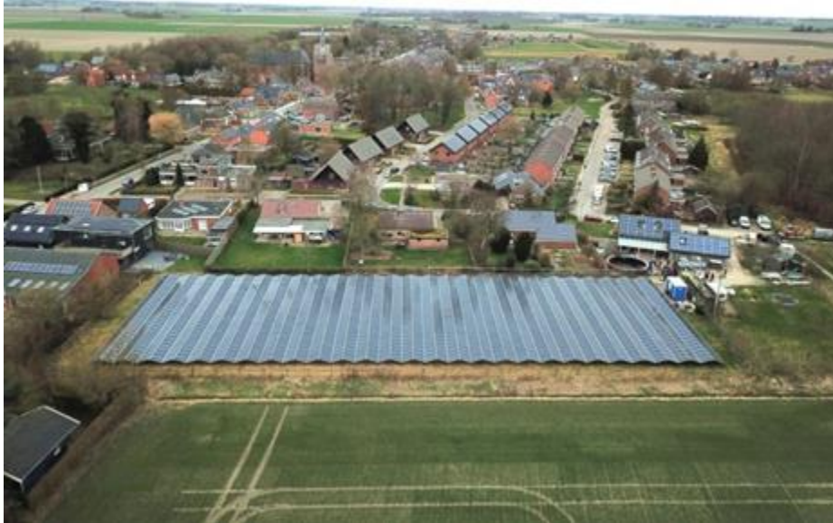
Figure A1. aerial photograph of the "Freek Sonneveld".
