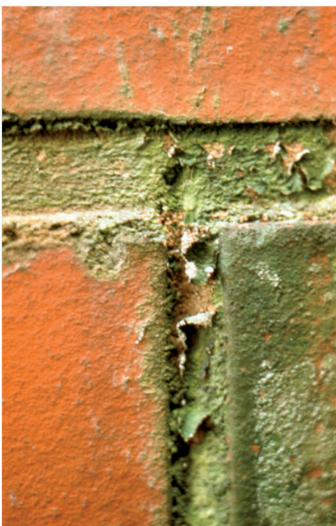
Figure 9. A macroscopically visible, curled up “biofilm-skin,” developing in an environmental biofilm on the mortar of a brick wall upon drying. The interaction between the EPS molecules and the sand grains in the mortar can become so strong that during the curling process, grains are pulled out of the mortar (Flemming 2008). Reproduced with permission of the publisher, Springer Int. Berlin, Heidelberg, Germany.
