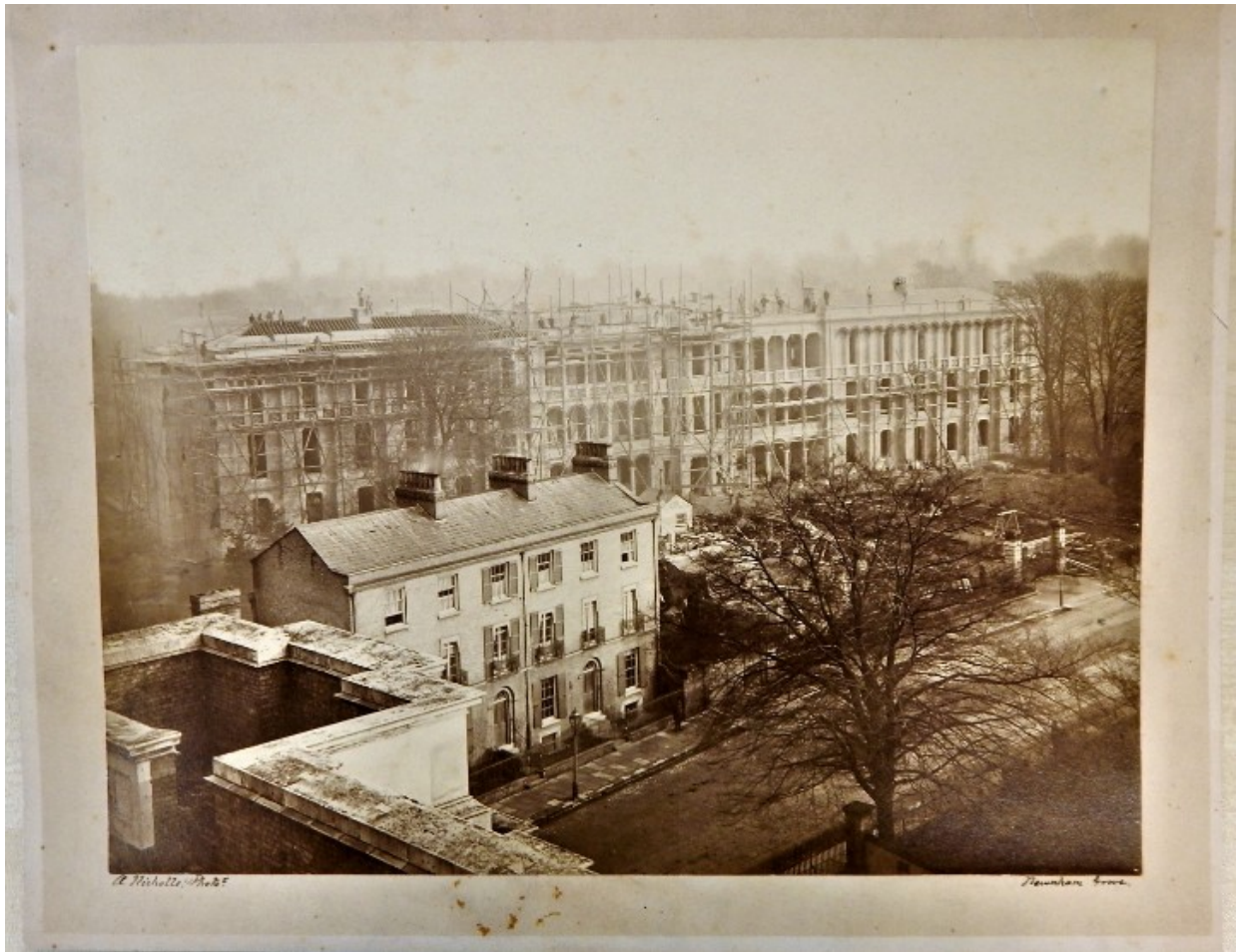
Figure 1.1 – Arthur Nicholls, The construction of Addenbrooke's Hospital, Cambridge. Cambridge Central Library Local Studies Collection– H.A. J63 7779.
