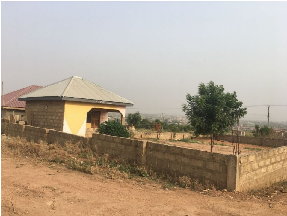
Figure 3. A compromised building built to protect the land /announce one’s physical presence on the land.
