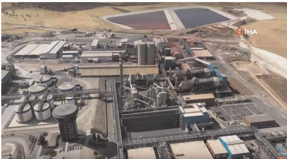
Figure 1. The 3D view of Mazıdağı, Mardin. EtiBakır Mazıdağı phosphoric acid, sulfuric acid, metal leaching, and metal electrowinning plants.
