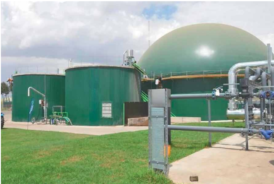
Figure 9. The Högdalen CHP-plant in Stockholm, Sweden [36].
