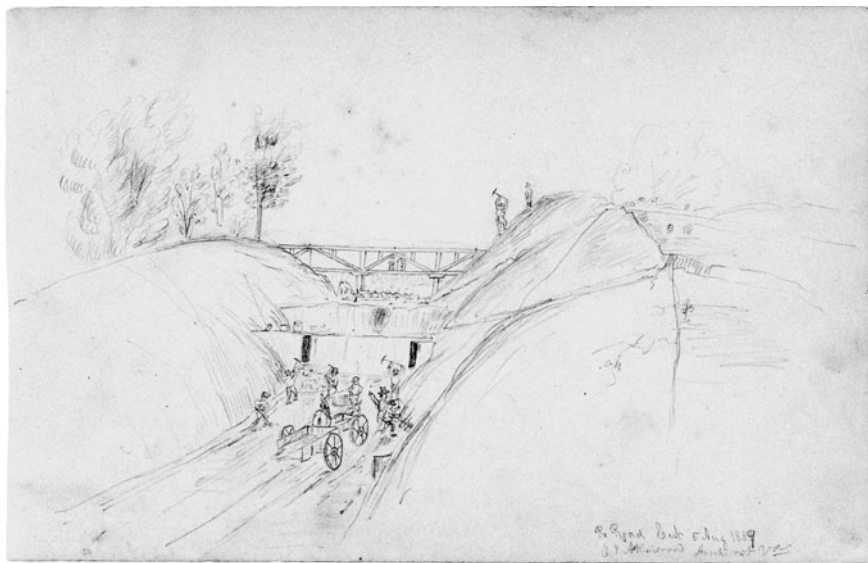
Figure 2. Laborers at work on a railroad cut on the Orange and Alexandria Railroad near Amherst, Virginia, in August 1859, as depicted in this image from the A. B. Petcolas drawing book. Workers strike at the sides of the cut with picks while horses wait to cart the earth away. Courtesy Virginia Historical Society, Richmond, Virginia.
