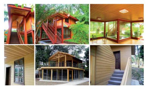
Figure 2. The applications of WPC in the indoor or outdoor ceilings and sidings.
