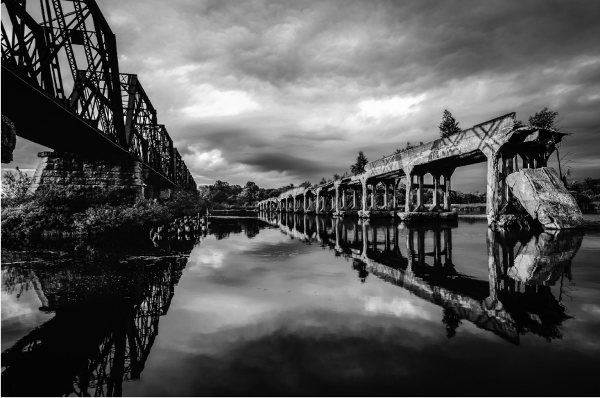
9.7 “American Ruins 2,” Escanaba, Michigan, 2011. On the left runs the Canadian National Railway bridge over the Escanaba River, one of only two historical lattice truss bridges in Michigan. The company removed and replaced the bridge in 2015. On the right, ruins of the Bay Shore Road bridge jut into the river. Delta County and the U.S. Army Corps of Engineers demolished this bridge in 2015. Photo by Lynne Heasley.
