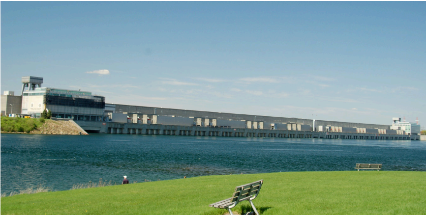
4.8 Robert Moses generating station. Photo by author.
