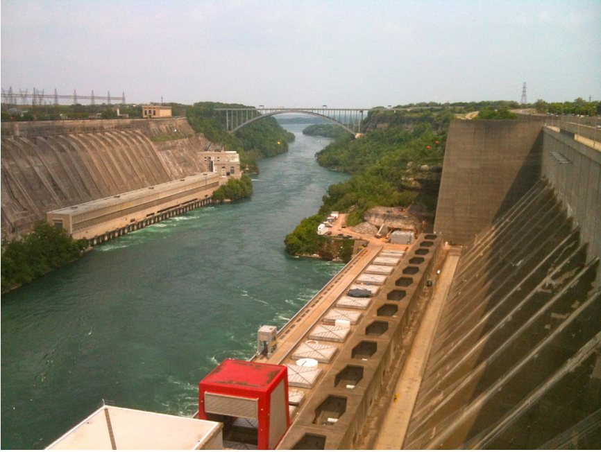
4.7 Moses and Beck power stations. Photo by author.
