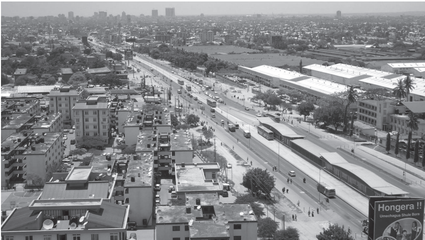
Figure 5.3 BRT Corridor in Dar es Salaam.
