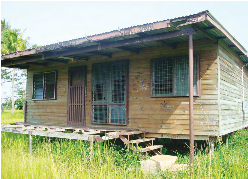
Figure 6.2 Abandoned government house at Nomad Station, 2013.
