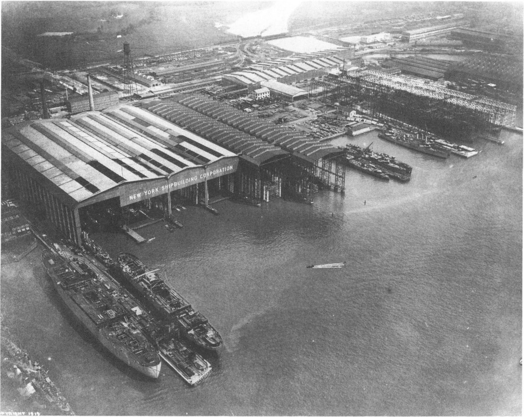
Aerial view of New York Ship, the world's largest shipyard, c. 1919. Note the original plant at left with a troopship outfitting. Note also the Clemson-class destroyers outfitting near the Middle Yard. National Archives
