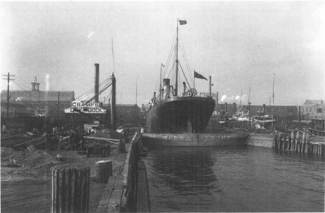
Cramp's dry dock, with British steamship Eagle Point docked for repairs, c. 1900. The caisson closing the dock was built at the shipyard. Library of Congress
