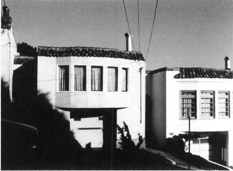
Figure 33. A two-module type, on Ridgewood, between Joost and Mangels, Westwood Highlands. The simplest configuration of modules that architect Strothoff orchestrated sets a narrow, recessed entrance module next to a broader module that includes shallow bow windows above a street-level garage. Variants of this type on streets that are less steep are somewhat more ample; fully detached, they are set further back from the street.
