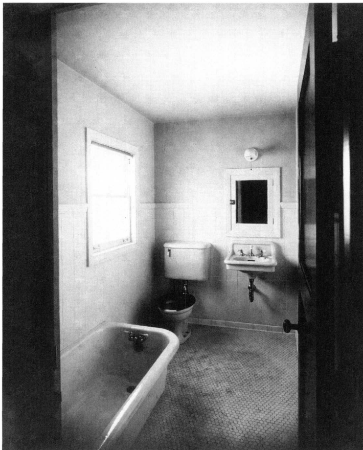
Figure 10. A typical bathroom ( above ) from the Ford Homes. Bathrooms, located on the second floor, used standardized fittings.
