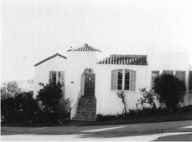
Figure 40. A corner house at intersection, Hazelwood and Brentwood, Westwood Highlands. Modular design allowed houses to be configured on unusual sites. This block ends in an acute angle and the house is pivoted dramatically to fit the space. The garage is located under the entrance module, but the garage doors are at a right angle to the entranceway, in the ell created by flipping the second window module so that it is perpendicular to the rest of the mass.
