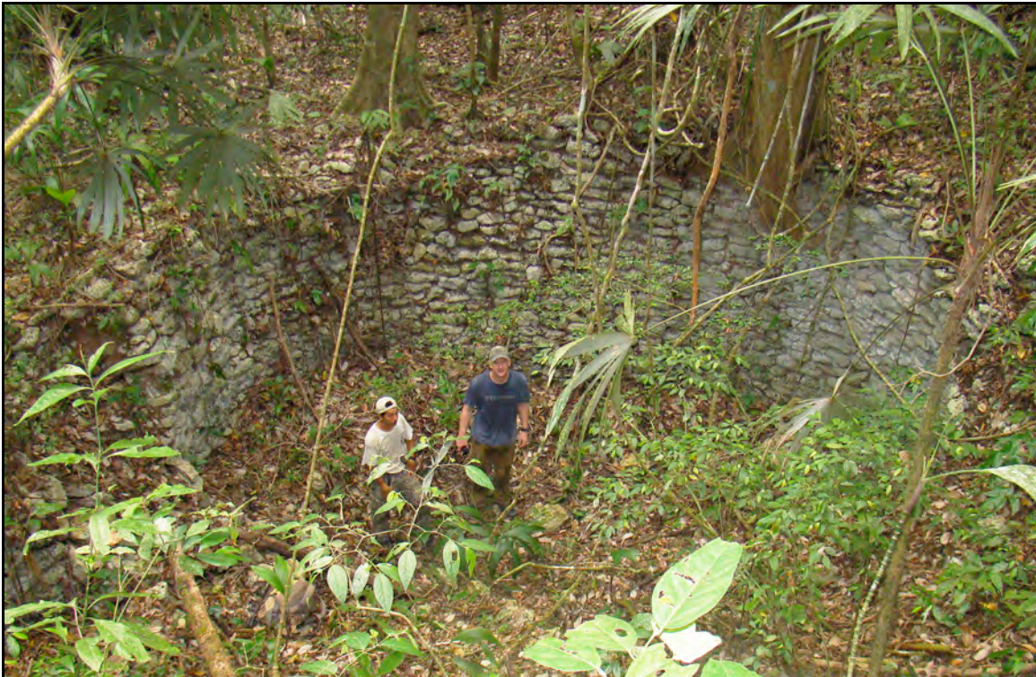
Figure 2.14. Photograph of masonry cistern at Tipan Chen Uitz, Cayo District, Belize (photograph by Christopher R. Andres).
