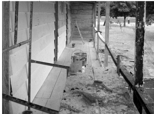
Figure 6. Scraping and repainting in the Catetinho veranda, first half of February, 2012. Supac digital archive.
