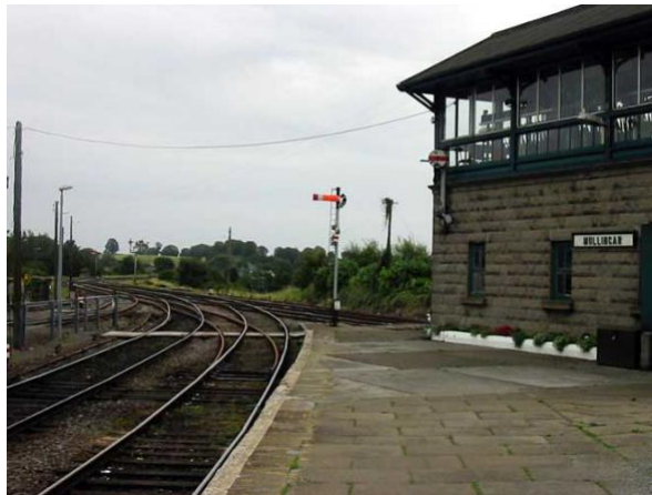
Figure 3. Mullingar Railway Station (author's photo, 2002).
