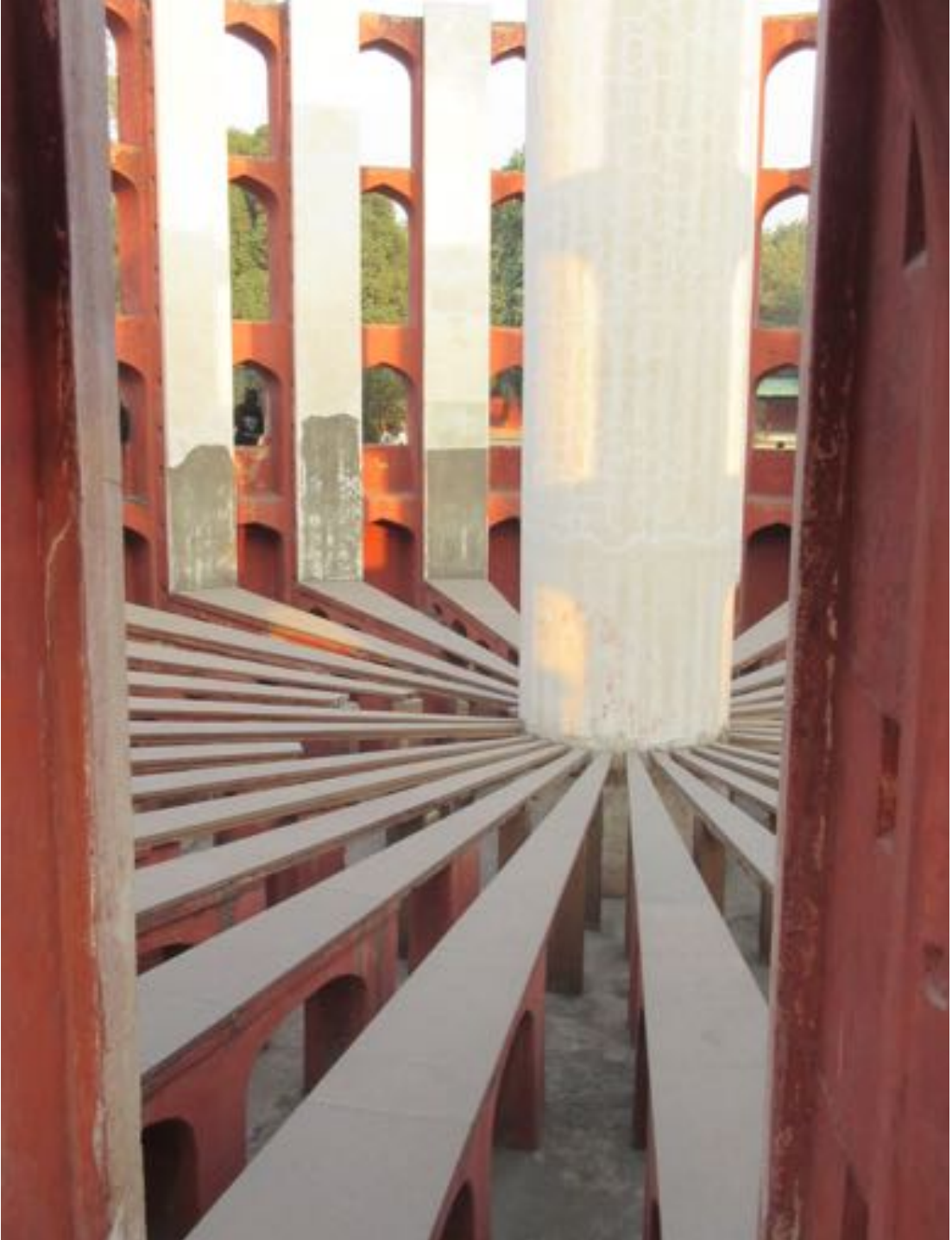
One of thirteen architectural instruments at Jantar Mantar, an astronomical observatory built of concrete in the 18th century, to predict the times and movements of the sun, moon, and planets. New Delhi, India (2016).
