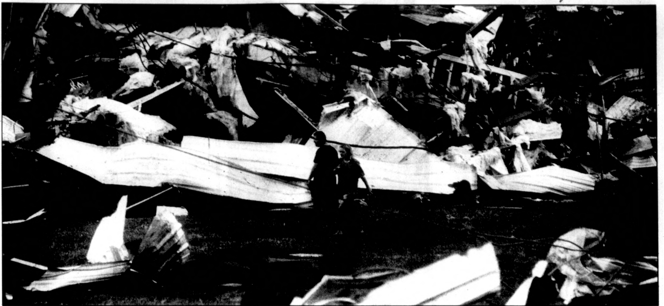
A man and woman examine the twisted wreckage of Glass Masters on U.S. 49 Frontage Road in Richland, Miss., shortly after it was destroyed by a tornado late Monday afternoon, April 28. With parts of the U.S. recovering from deadly tornadoes, more heavy storms are making their way across the South.
