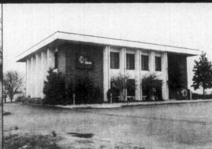
North Banking Center, 1104 Chestnut Street
