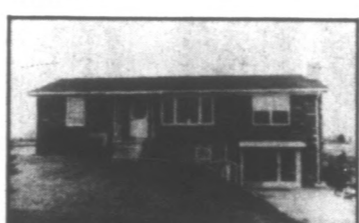
Brick 4 bedroom home with over 3,000 sq. ft. under roof. Relax this summer in your own swimming pool and hot tub. $80,000.
