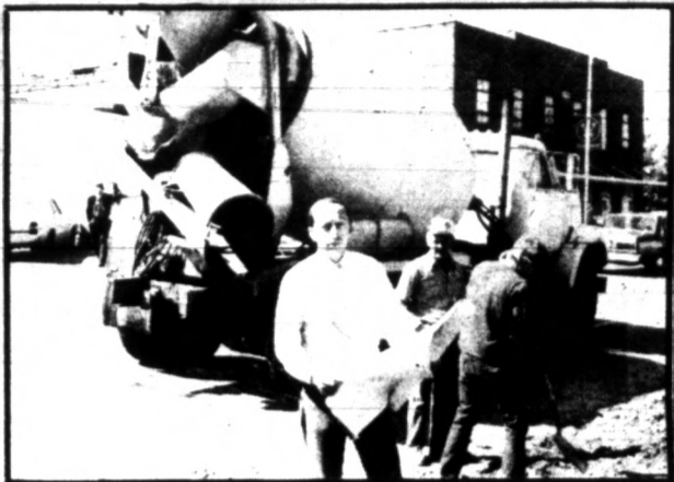
Street repair and renovation
