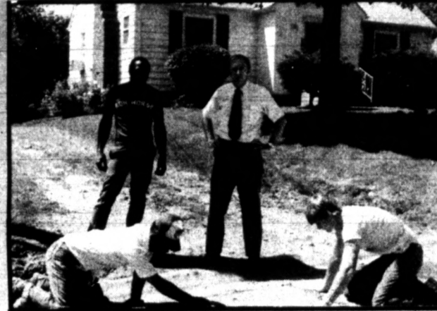
Sidewalk repair and renovation
