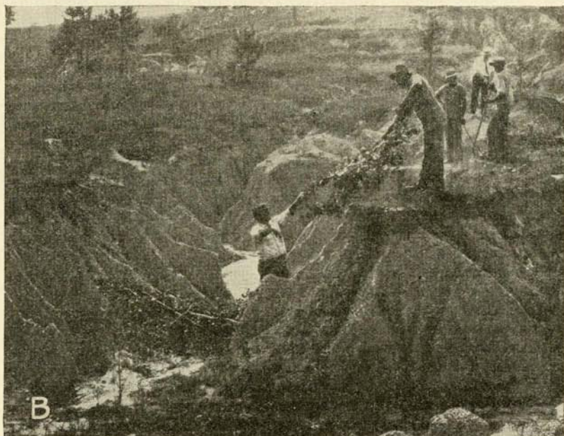
FIGURE 2.—Treatment given a gully preparatory to planting black locust or other vegetation: A, Plowing in the gully edges. Intervening areas between the gullies should also be deeply plowed. B, Constructing the proper type of dam
