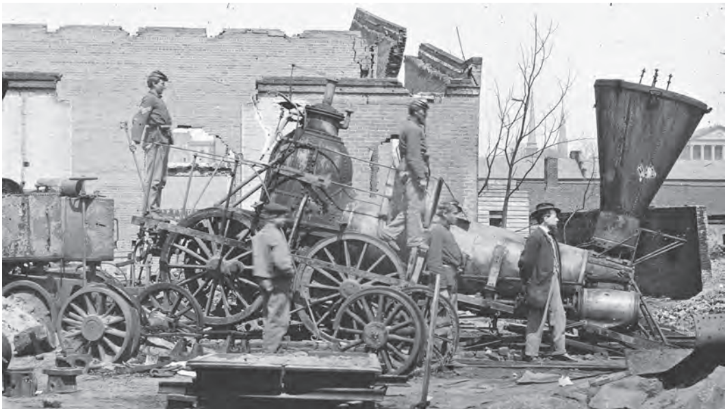
War brought destruction across the South. Governmental and private buildings, communication systems, the economy, and transportation infrastructure were all debilitated. Richmond, Va. Crippled locomotive, Richmond & Petersburg Railroad depot, c. 1865. Library of Congress.
