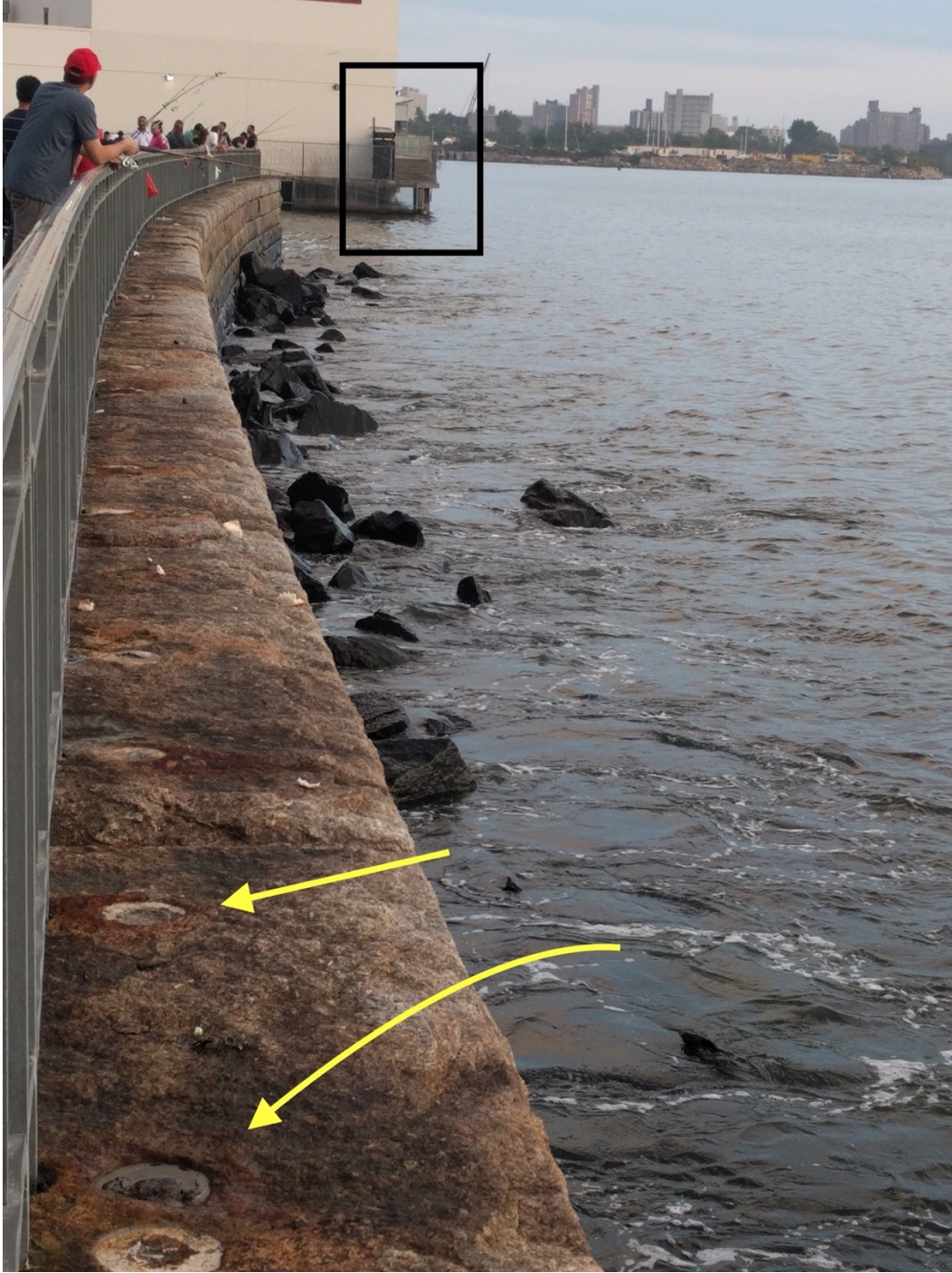
Figure 18: Recreational Fishing in Gravesend Bay. The area in the black box is a ledge that was formerly open for crabbing and is now closed for storm surge risk. The large building in the top left corner is part of Ceasar's Bay Bazaar (a shopping complex). The horizon shows housing complexes in Coney Island. The yellow arrows point to large holes in the sea wall from the original damaged, rusted fencing. Photo by Rose Jimenez 2018.
