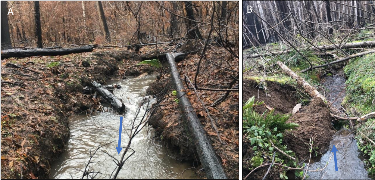
Figure A16. Examples of recent bank collapse in SWP from (A) Dec-20 and (B) Mar-22. Blue arrows indicate flow direction.
