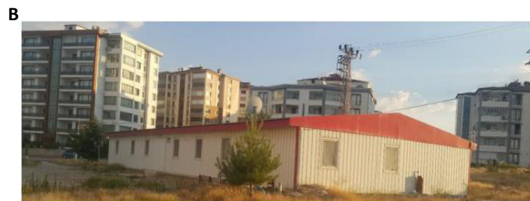
Figure 2. System installation location. A: Location of the office building; B: Office building of which passive cooling is done.
