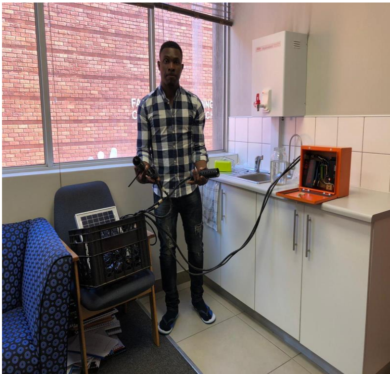
Figure 6.7: MISRA v1.1 Full Setup with Solar Panel
