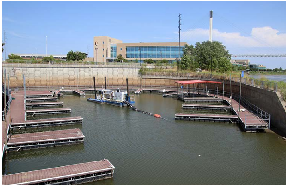
Figure 35: Image of the marina being dredged in August 2022. Sediment is still visibly exposed under the docks on the right side. Part of the Bob Kerry Bridge is visible in upper right corner.
