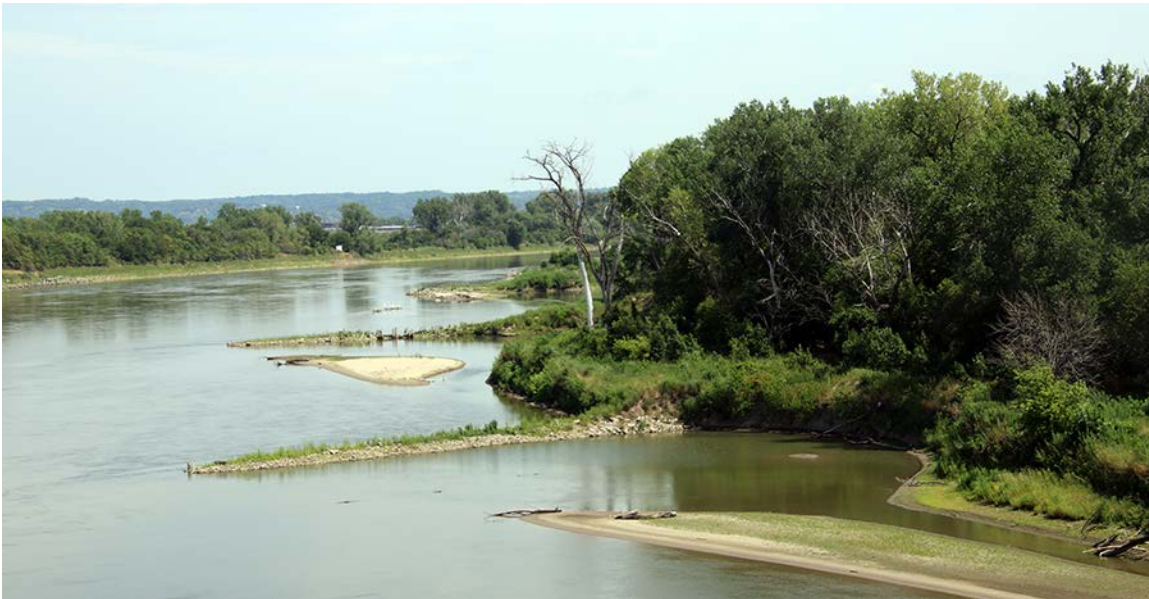
Figure 35: View looking upstream at Iowa side of the river showing the prominent wing dikes with eddy scour pools immediately downstream and sand bars further downstream. This image was taken during August of 2022 when flows were relatively low and the wing dikes and associated features well exposed.
