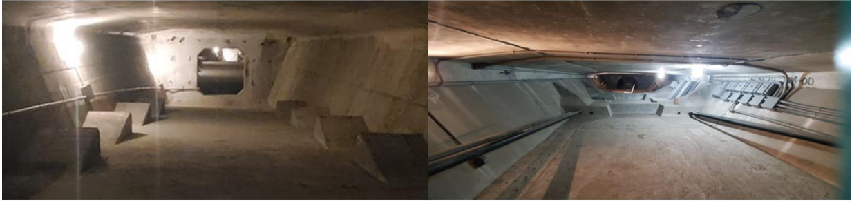
Figure 3: Seabreeze Bridge (Left), Broadway Bridge (Right)
