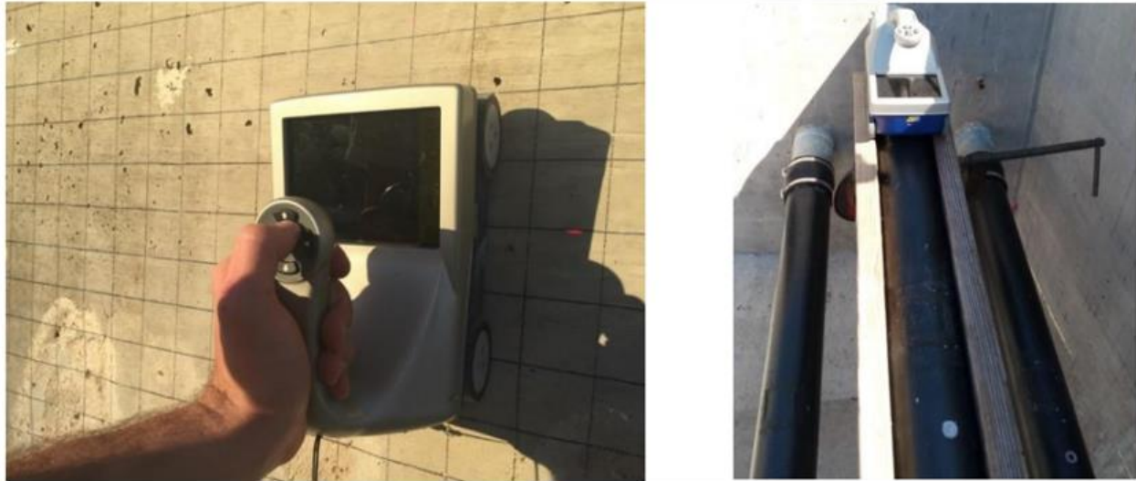
Figure 7: StructureScan Mini HR GPR unit (Left), GPR unit inspecting the external tendons (Right) (Hurlebaus, Hueste, Karthik, and Terzioglu, 2016)
