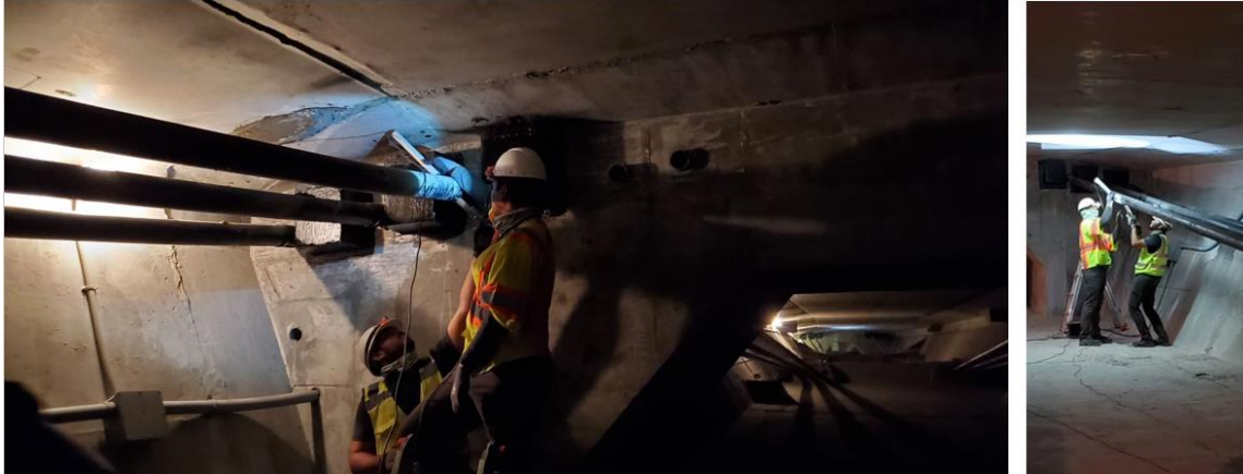
Figure 19: Ultrasonic Pulse Velocity (UPV) Testing
