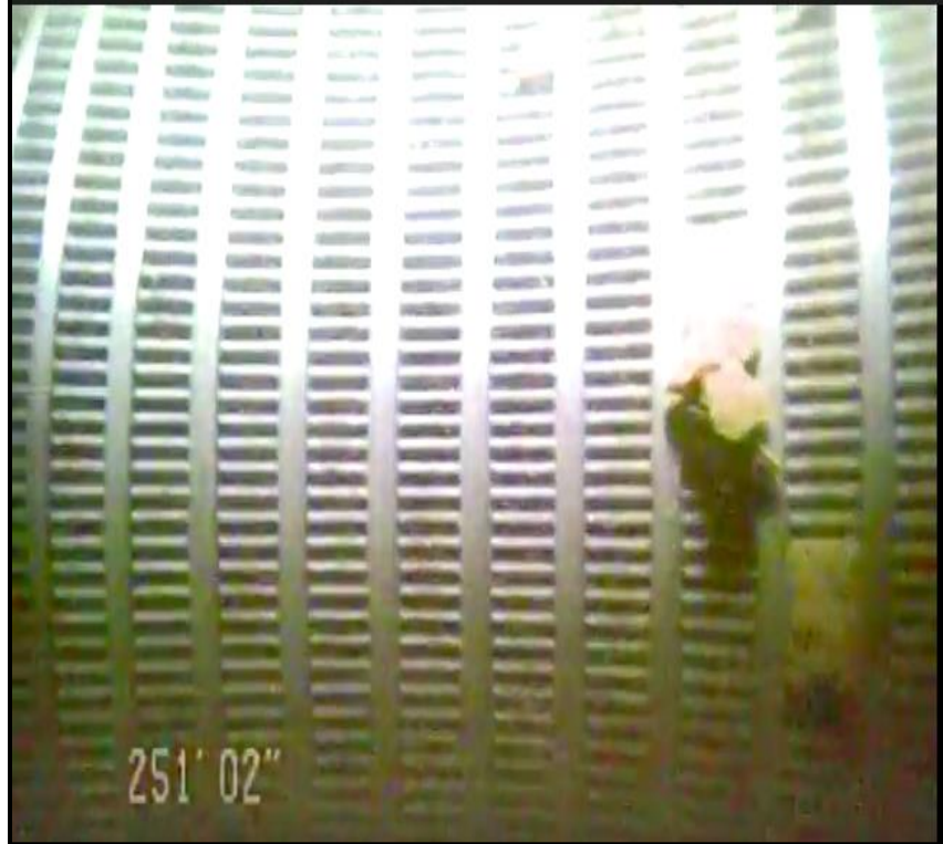
e. Well screen mechanically scrubbed October 2017
