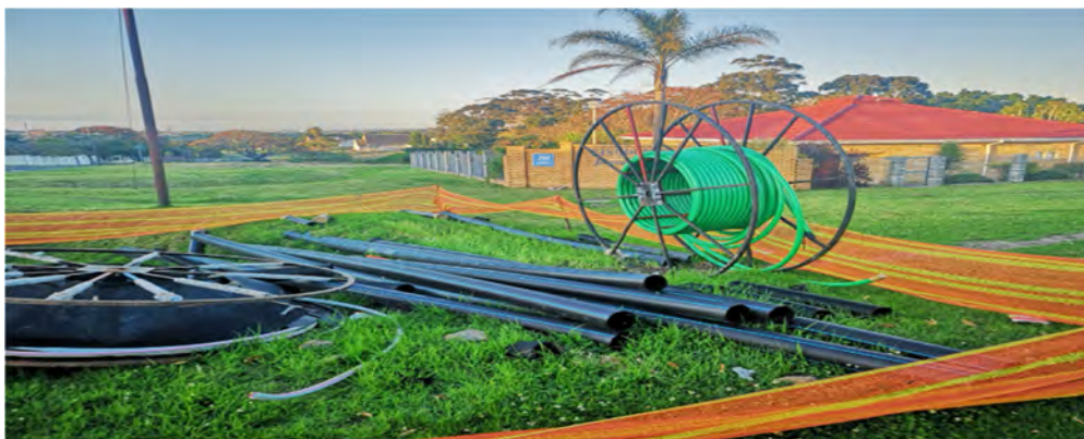
Figure 8-1: Installation of optic fiber, Cambridge, East London, South Africa (Nov 2019)
