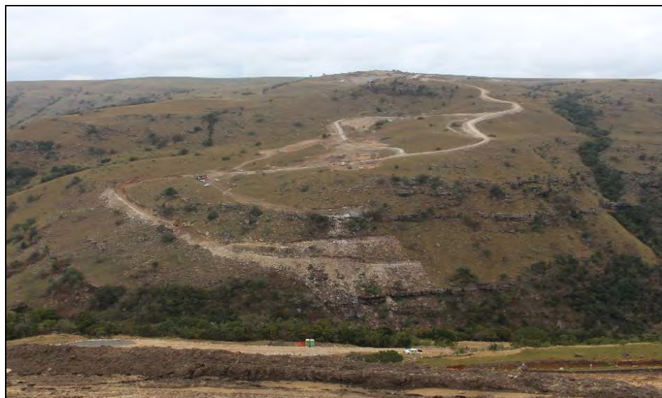
Figure 8.5: The abandoned bridge site at Mtentu following amaDiba protests and the withdrawal of Aveng Strabag from the project (D. de Villiers, 2020)
