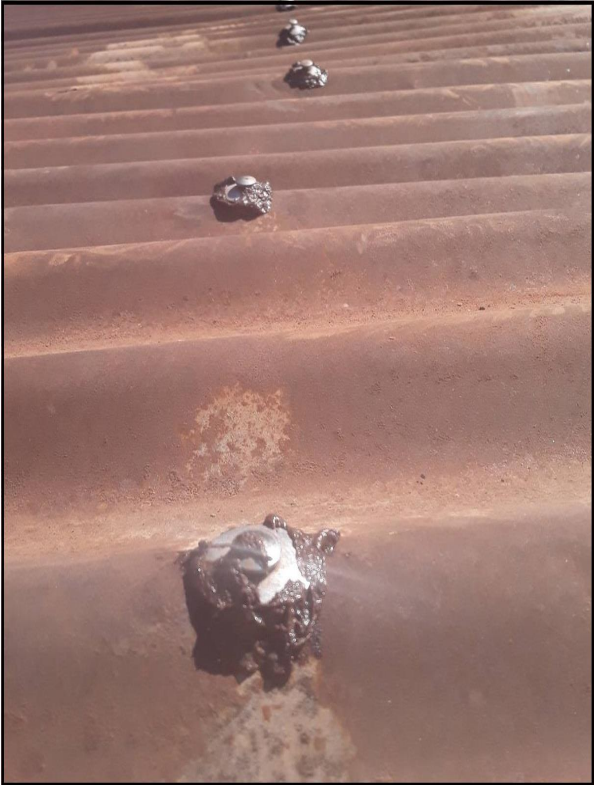
Figure 4.5: Use of birdlime in roof waterproofing
