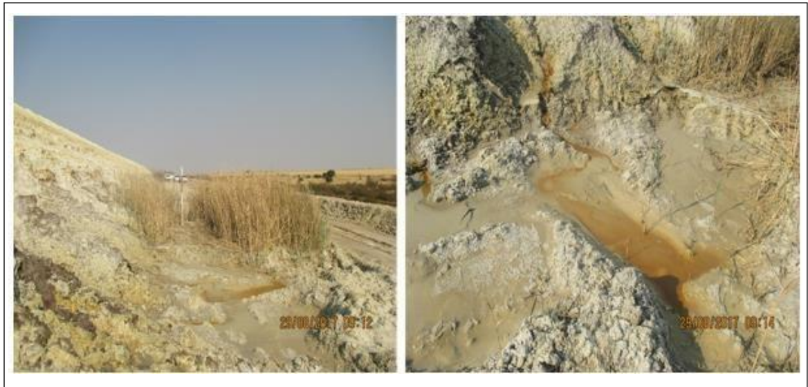
Photograph 2: Pictures that were taken at the foot of the FSSW8 tailings dam. The pictures indicate evidence of visible water on surface and increased vegetation growth at the foot of the dam.
