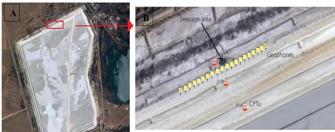
Figure 6.1: (a) Aerial view of the tailings dam where the seismic stations were installed. (b) Zoomed in picture of figure 6(a) showing the distribution of the seismic stations on the tailings dam and the location of the cone penetration tests. The area with seepage is also indicated in the picture.
