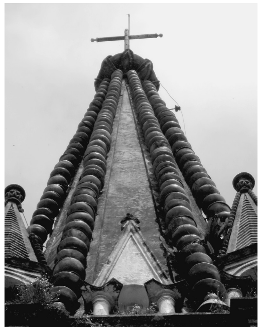
FIGURE 14. View of the spire of El Santuario de Guadalupe, showing how its clay pots diminish in size toward the top. Photo by author.
