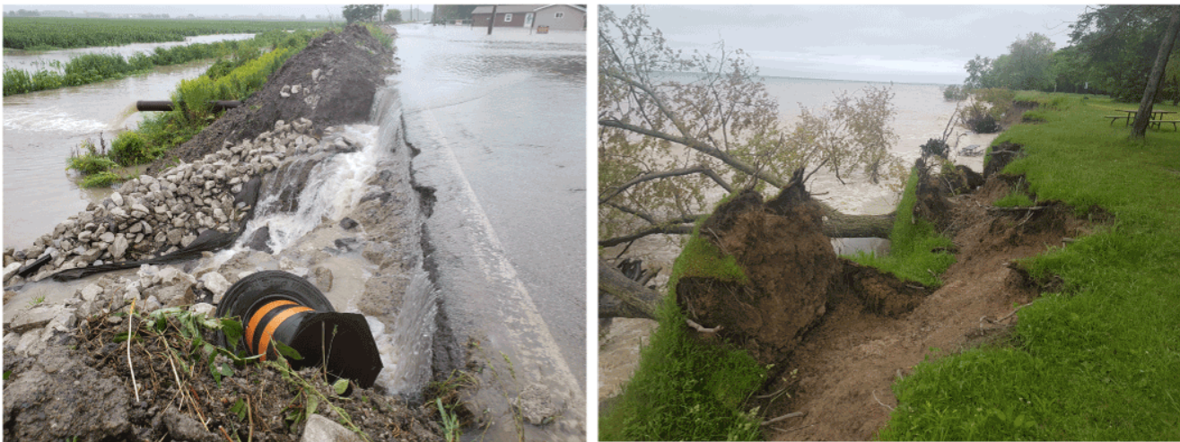
Figure 3.11: Left: Eroding bluffs along Lake Erie at Wheatley Provincial Park in 2018. Right: August 27, 2019 flooding at Erie Shore Drive. Increased shoreline erosion and flood risk are attributed to changes in lake levels, ice cover and exposure to wave energy. Source: Zuzek, 2020.
