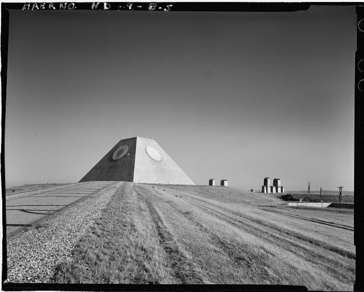
Figure 1: Missile Site Radar at the Mickelson Safeguard Complex near Grand Forks, North Dakota. | "5. Distant view of west oblique of missile site control building. To right can be seen intake and exhaust of MSRPP, on far right is accessway - Stanley R. Mickelsen Safeguard Complex, Missile Site Control Building, Northeast of Tactical Road; southeast of Tactical Road South, Nekoma, Cavalier County, ND", Benjamin Halperin, Library of Congress, https://www.loc.gov/pictures/item/nd0046.photos.199338p/ .
