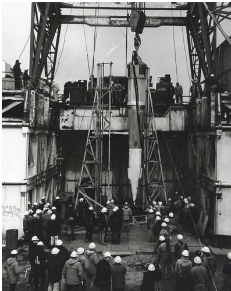
Figure 12: The Cannikin Device, containing the W-71 warhead, which was lowered into a nearly two-kilometer-deep shaft to be tested on Amchitka Island, Alaska. | Courtesy of Los Alamos National Laboratory Archives, https://farm9.staticflickr.com/8430/7597458904_385f8106ed.jpg .
