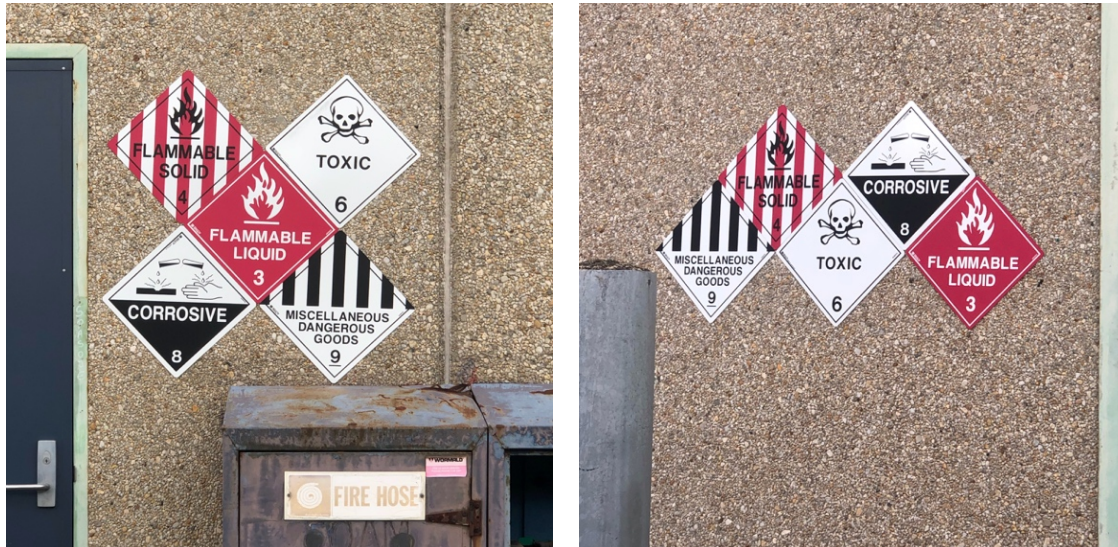
Figure 75. Hazard signs at a paint factory.
