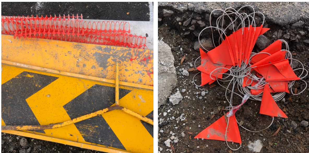
Figure 84. Traces of work conducted on my street during the first half of 2021.
