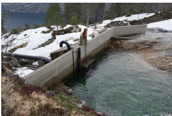
(a) Grønhaug plant intake dam area
