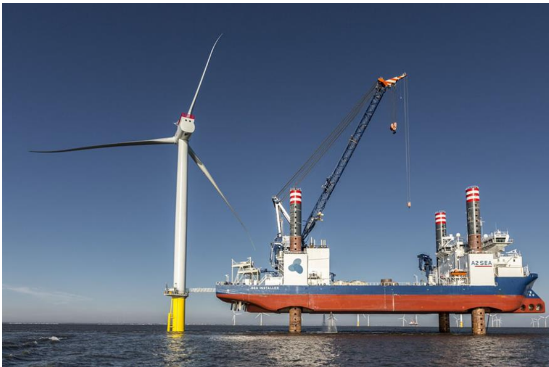
Figure 4.2: The figure (Shaun Campbell, 2014) shows a lifting operation
