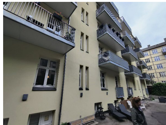
Figure 6. Tårnborgvej, SAVE-value 4, EPC label C. Left: The front facade, restored to its original look. Right: The rear façade, externally insulated.
