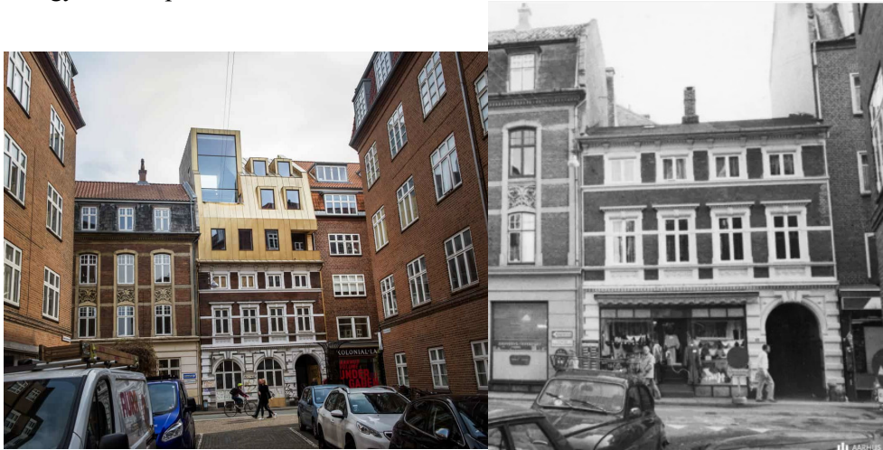
Figure 7. Mejlgade. SAVE-value 2, EPC-label C. Right: The present building with three new floors added. Right: The original building before the renovation.
